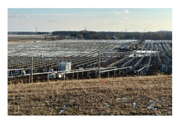
We've also installed 40% of the piles, the metal posts that support the solar arrays, and we've completed nearly 22% of the tracking system. This involves racking that goes across piles horizontally to hold the panels, and motors that allow the panels to rotate with the sun.
