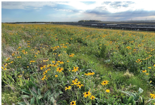
Pollinator field at our North Rock Solar Project
