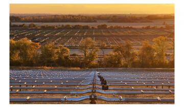
As we install the panels, we continue to install the DC cable that carries electricity from the panels to the inverter boxes. We've already installed the underground AC cable that brings electricity from the inverters to the substation.
