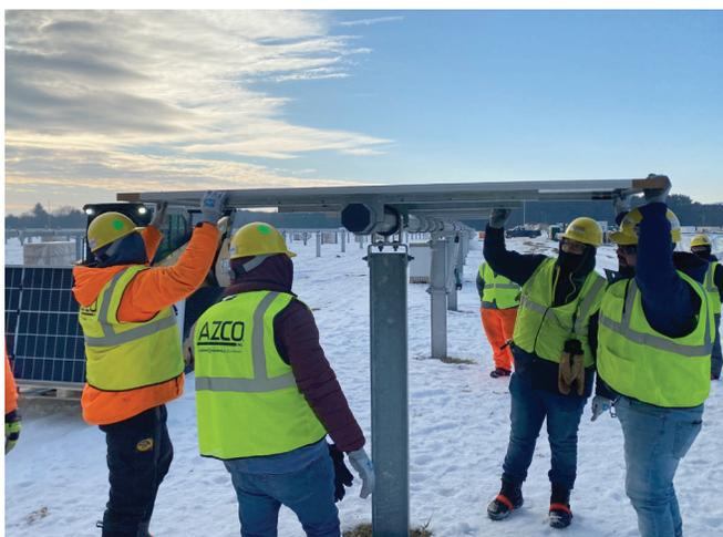
Installation of piles, the metal posts that support the solar arrays, is 100% complete, with the tracking system installation in progress. Racking goes across piles horizontally to hold the solar panels, and then trackers, or motors, rotate the panels with the sun. As of mid-January, tracking system installation is nearly 50% complete.
