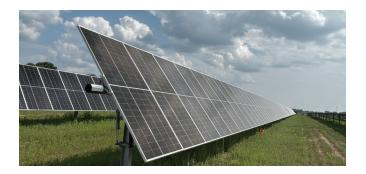
across piles horizontally to hold solar panels; trackers, or motors, are the components that rotate panels with the sun. As of early September, tracking system installation is 100% complete as well, and we've installed approximately 60% of the solar panels.
