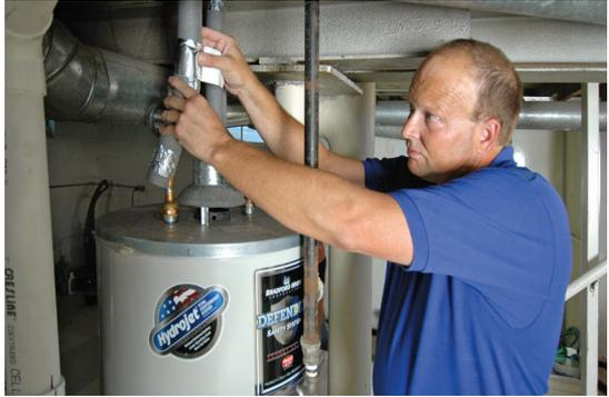
The tank wrap is a thick fiberglass blanket, secured around the tank by waterproof tape. Before installing any water heater insulation, shut off the power to the unit. When installing tank wrap, follow the manufacturer's directions exactly to ensure maximum efficiency, and be sure to leave these areas uncovered:
