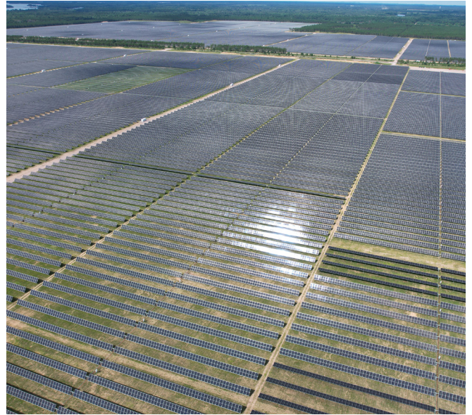
Completed Wood County Solar Project
