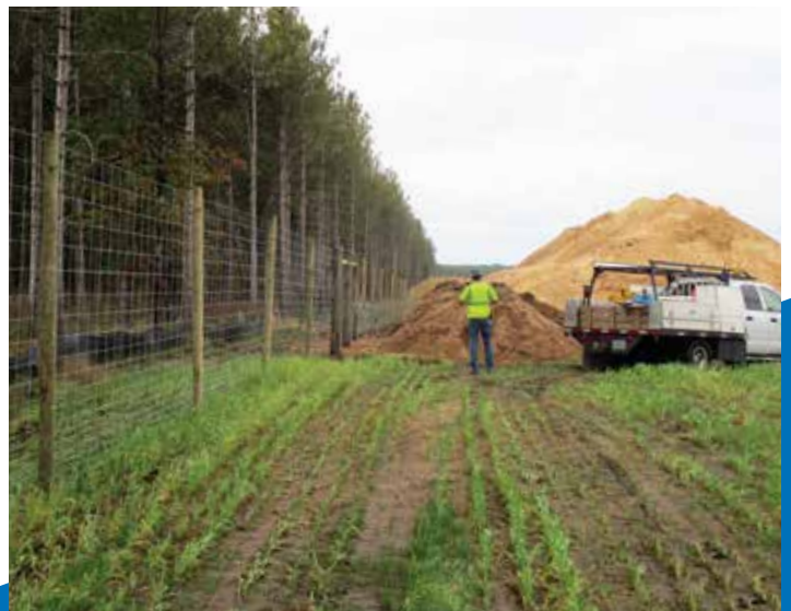
Fence installation on the west project boundary
