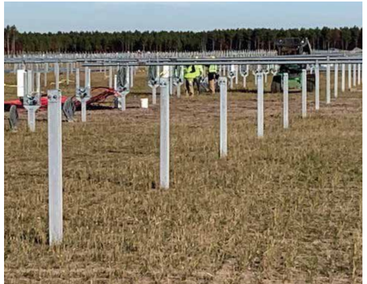
Crews install the solar racking system
