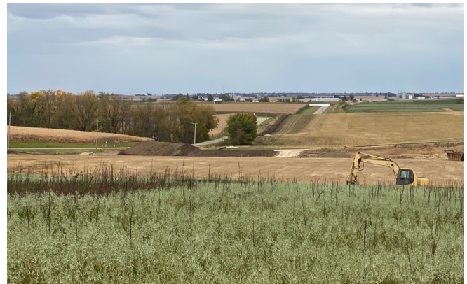
Crews install access roads at the Grant County Solar Project.
