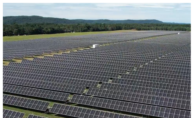
The final look of a solar project once complete (Bear Creek Solar Project, Richland County, WI).
